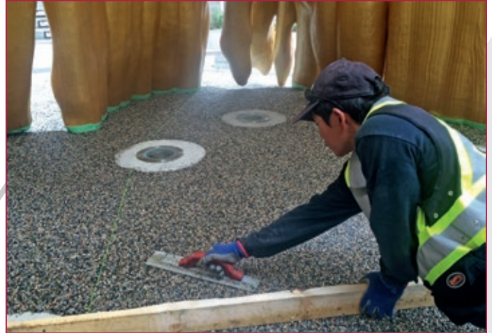
Gut verdichten | Good compacting
